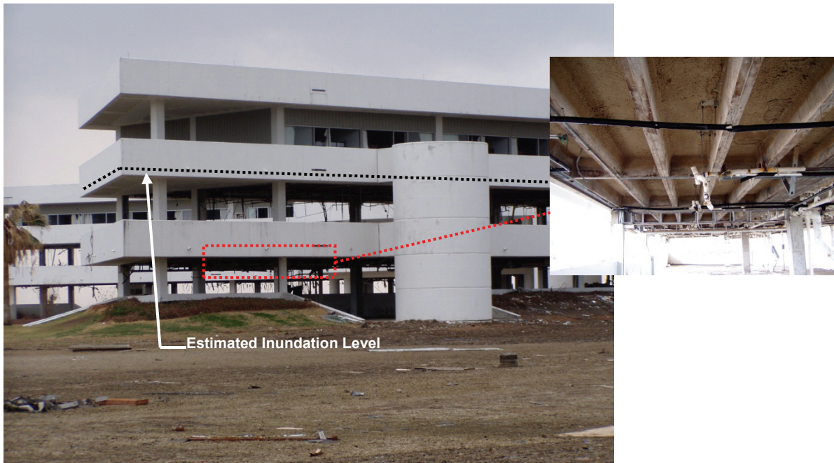
Figure 2-31 Pass Christian office building with cast-in-place concrete pan joist floor system that suffered non-structural damage at first two floors but no structural damage (Hurricane Katrina, 2005).
