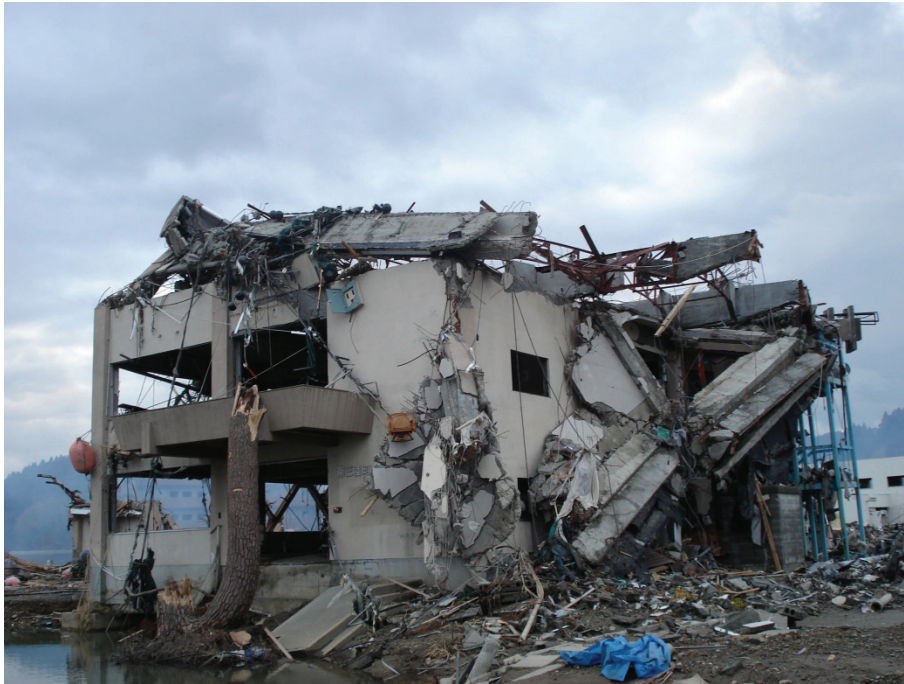
Figure 2-27 Collapsed top floor of reinforced concrete building with steel truss roof (photo courtesy of I. Nistor, ASCE, 2012).
