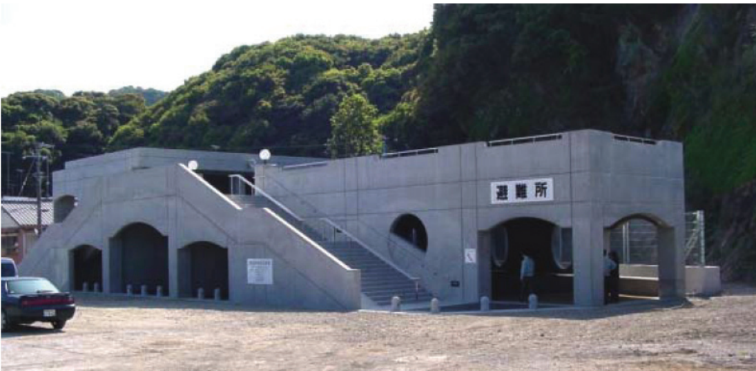
Figure A-5 Tsunami refuge in Kaifu, Japan.
