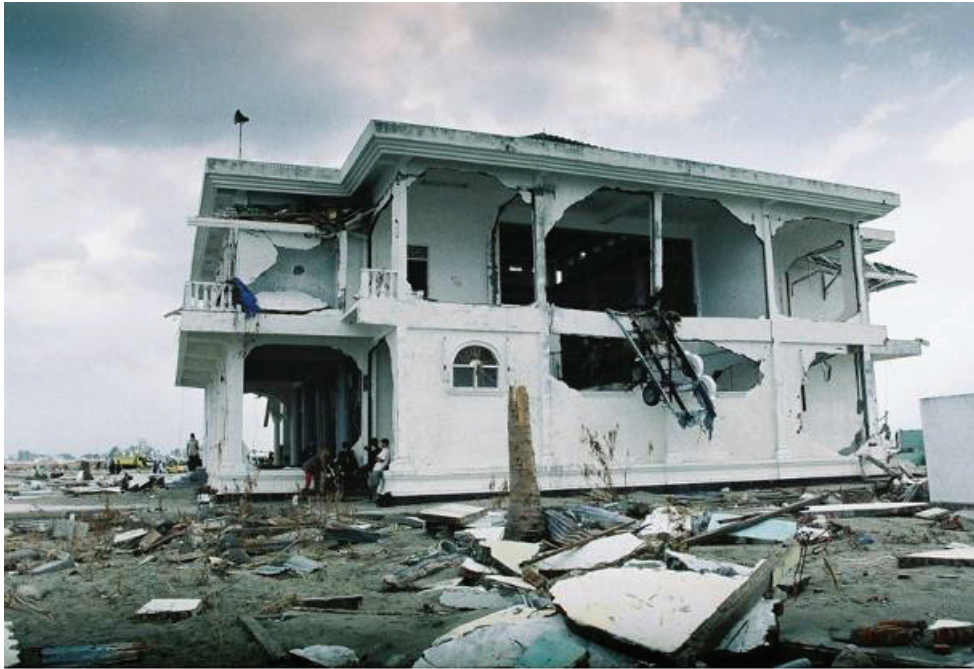
Figure 2-15 Example of surviving reinforced concrete mosque in Uleele, Banda Aceh (photo courtesy J. Borerro).
