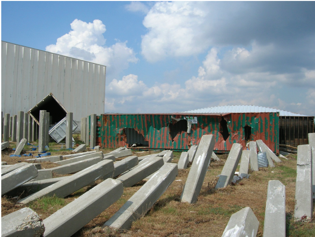
Figure 2-33 Failure of prestressed piles due to damming effect of shipping container (Hurricane Katrina, 2005).
