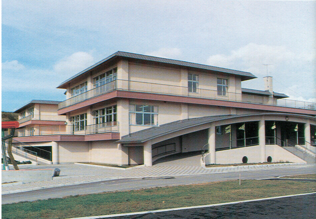
Figure A-7 Aonae Elementary School. Upper floor is intended for use as tsunami refuge space.
