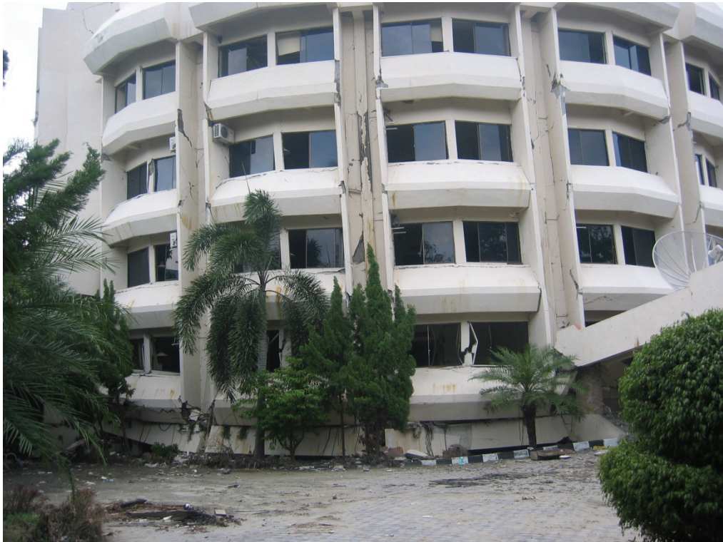
(b) Soft story failure
