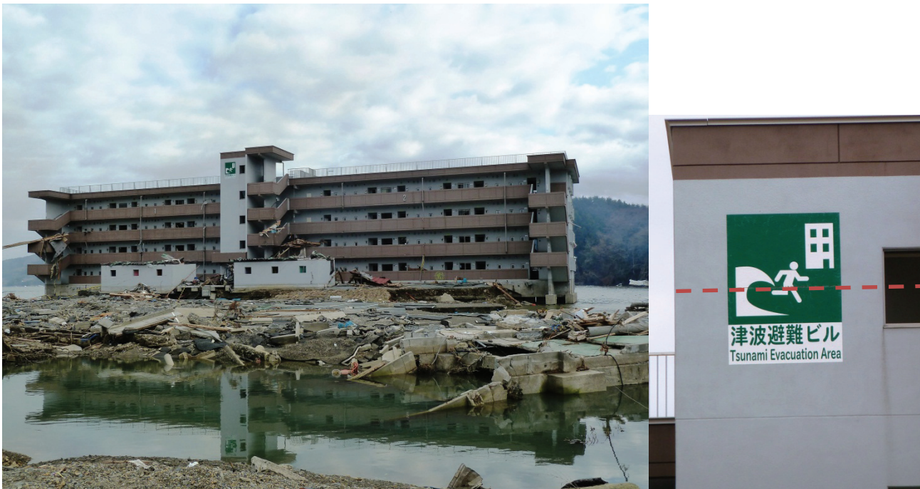
Figure 2-23 Minamisanriku designated coastal evacuation building – note tsunami trace on sign (photo courtesy of I. Robertson, ASCE, 2012).
