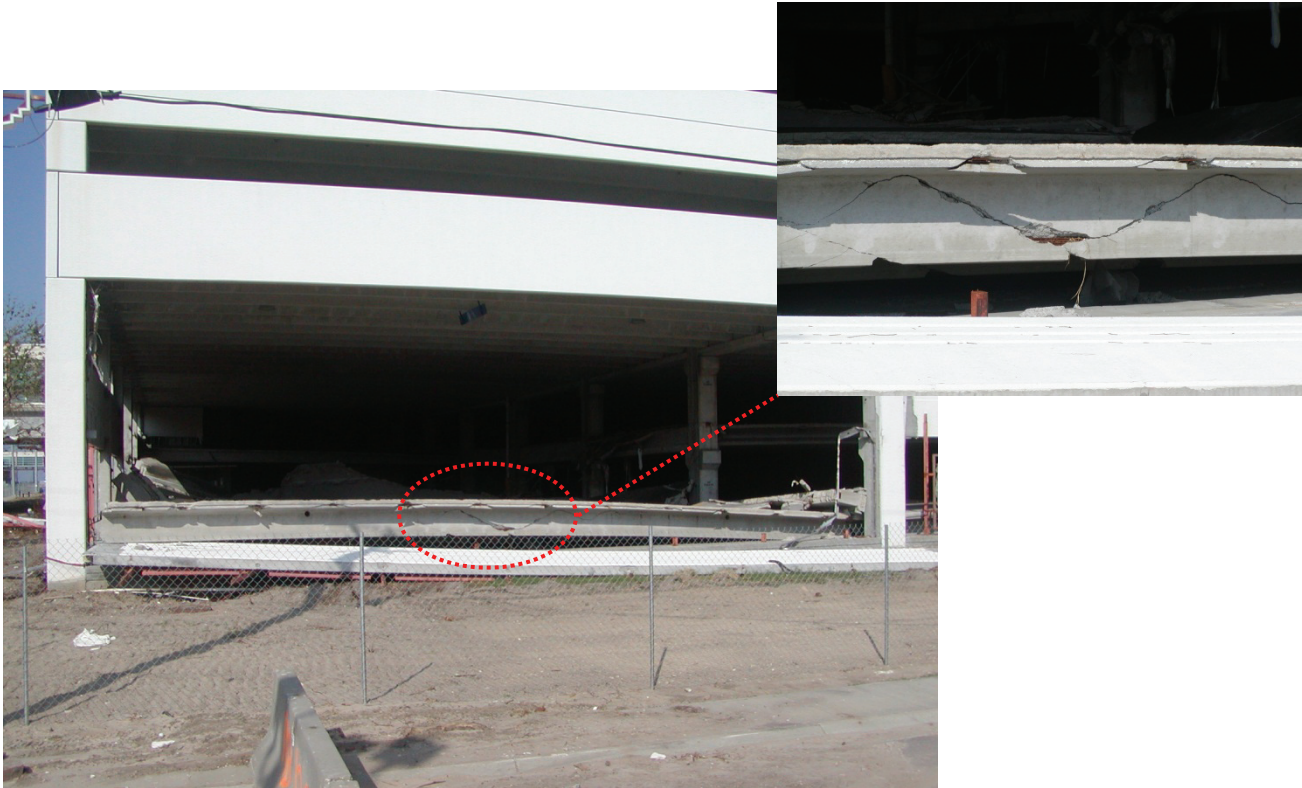
Figure 2-34 Negative bending failure of a prestressed double-tee floor system due to uplift forces (Hurricane Katrina, 2005).
