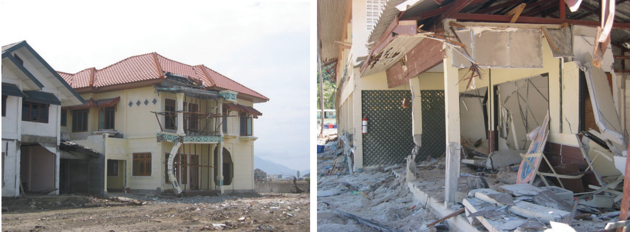
Figure 2-17 Damage to non-engineered concrete columns due to debris impact (photos courtesy of M. Saatcioglu, A. Ghojarah and I. Nistor, CAEE, 2005).
