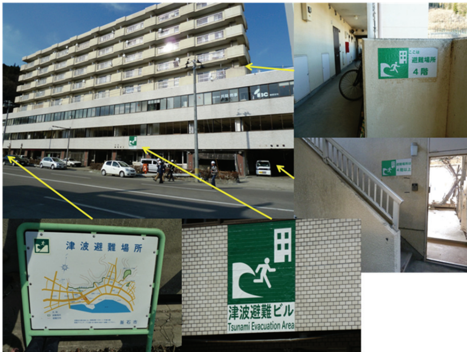
Figure 4-5 Residential apartment building in Kamaishi, Japan, with designated refuge area at or above the fourth level.
