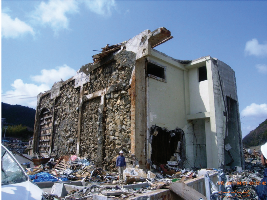
Figure 2-28 Overturned cold storage building in Onagawa (photo courtesy of G. Chock, ASCE, 2012).
