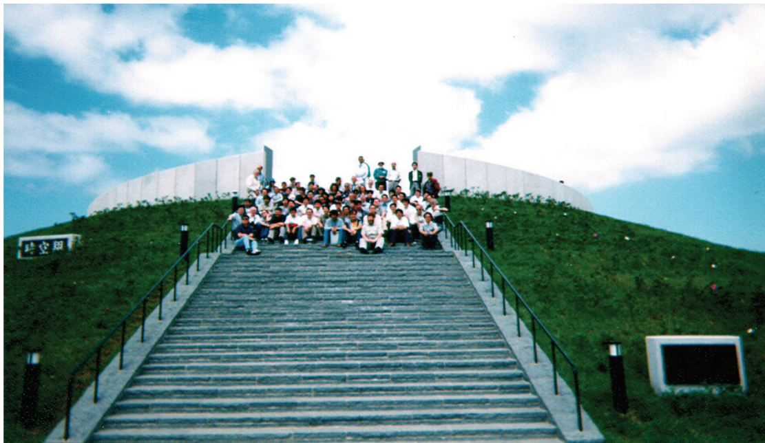
Figure A-6 Berm constructed for tsunami refuge in Aonae, Japan.
