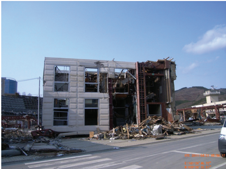
Figure 2-29 Overturned steel-framed office building in Onagawa (photo courtesy of G. Chock, ASCE, 2012).
