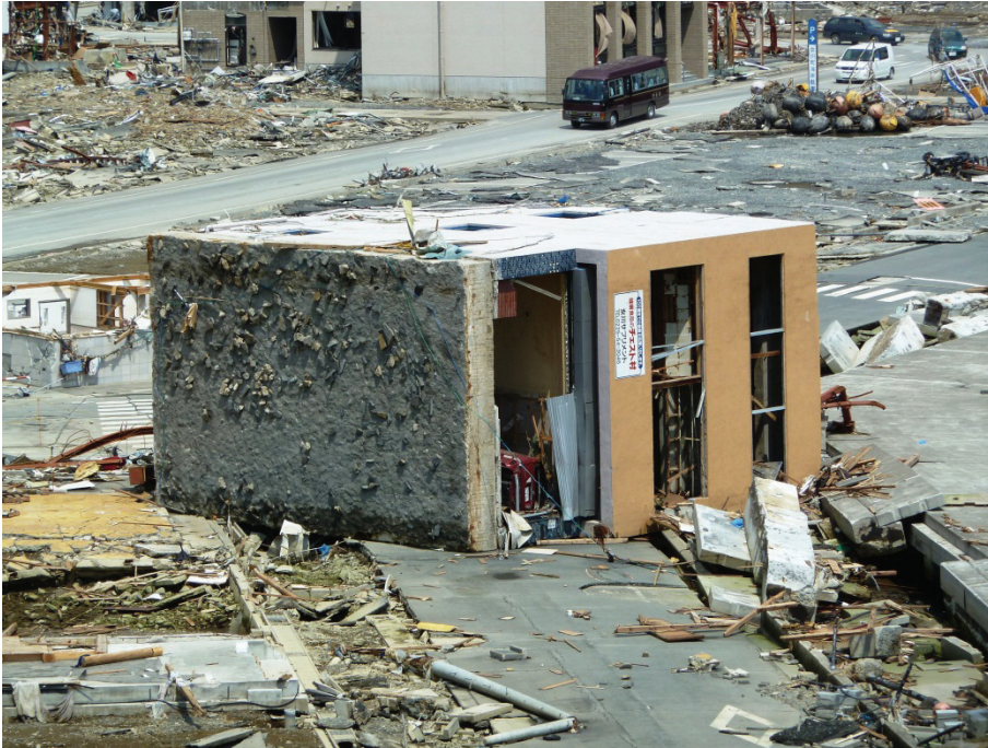
Figure 2-30 Overturned three-story commercial building on mat foundation (photo courtesy of I. Robertson, ASCE, 2012).
