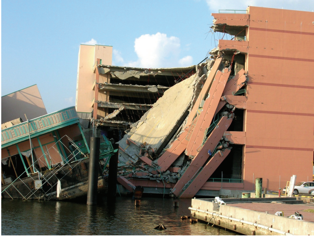
Figure 2-32 Progressive collapse of upper floors of a parking garage due to damage in lower level columns from impact of an adjacent barge-mounted casino (Hurricane Katrina, 2005).
