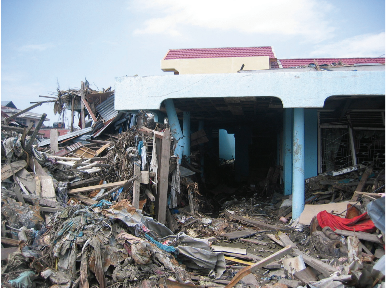
Figure 2-18 Damage to corner column due to debris damming (photo courtesy of M. Saatcioglu, A. Ghojarah and I. Nistor, CAEE, 2005).
