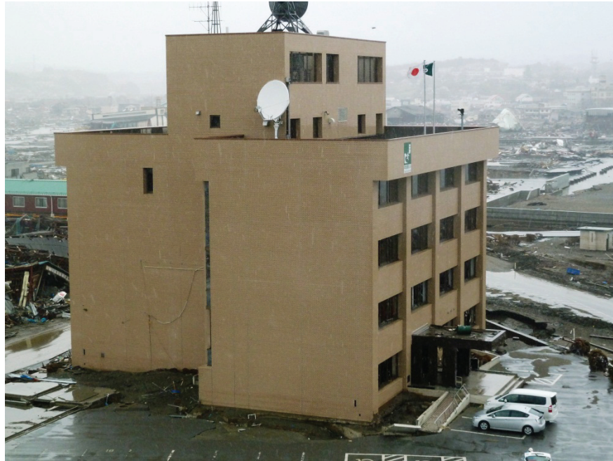
Figure A-1 Successful designated vertical evacuation building in Kesenuma Port, Japan.
