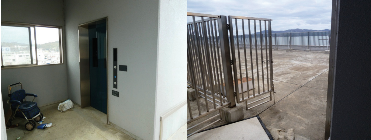
Figure 2-24 Exterior elevator and stairway access to large roof evacuation area protected by 2 meter high braced guard fence on Minamisanriku coastal evacuation building (photo courtesy of I. Robertson, ASCE, 2012).
