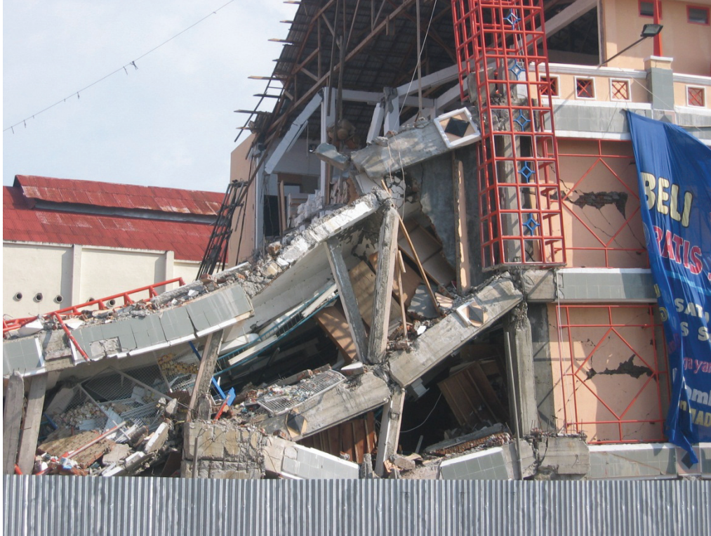
(a) Beam-column connection failures
