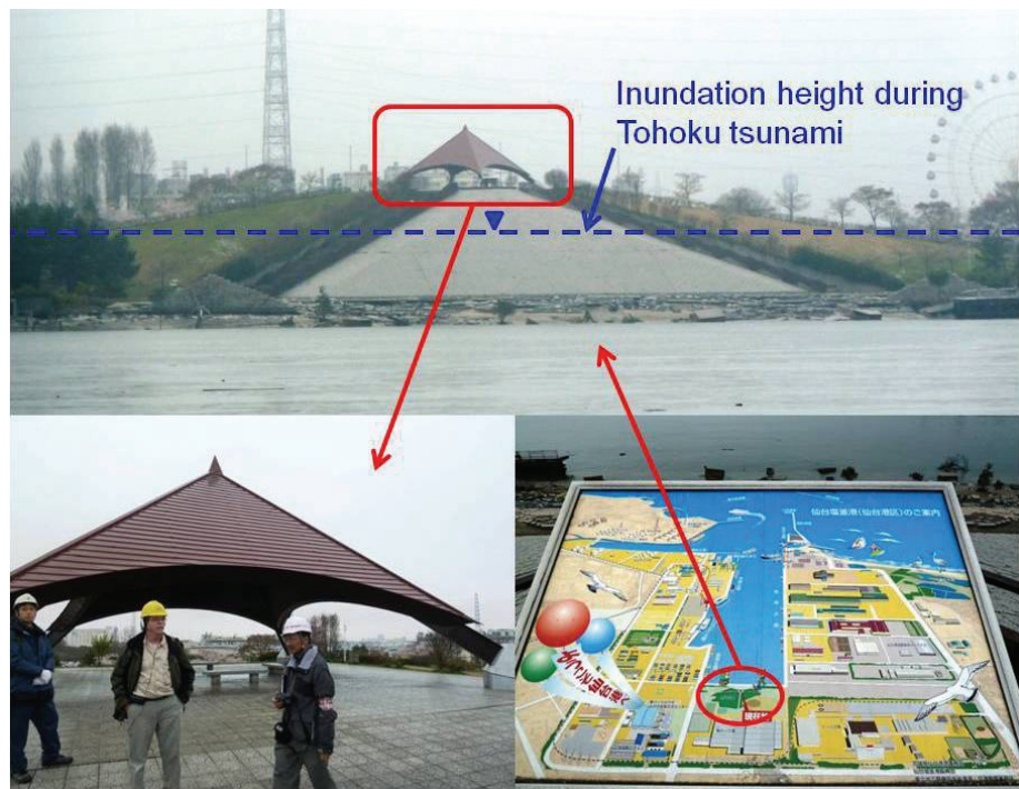
Figure 4-1 Soil berm combined with a community park at Sendai Port, Japan. Concrete lining on the ocean face can deflect incoming waves while sloped sides provide for quick access. Graphic in the lower right side illustrates where the evacuation berm is located in Sendai Port.
