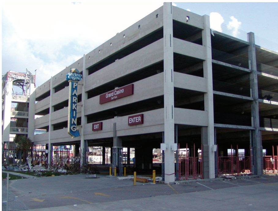
Figure 4-2 Cast-in-place reinforced concrete parking garage in Biloxi, Mississippi after Hurricane Katrina. Open structural systems allow water to pass through with minimal resistance, and interior ramps allow for easy ingress and vertical circulation.
