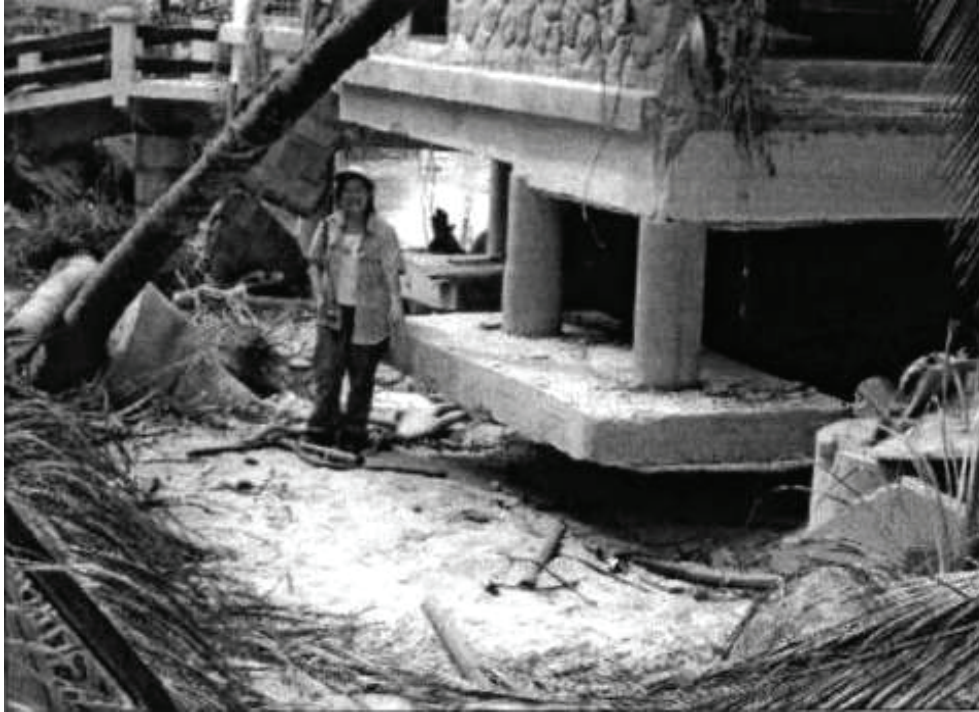
Figure 2-19 Scour around shallow spread footing in Khao Lak area (Dalrymple and Kriebel, 2005).
