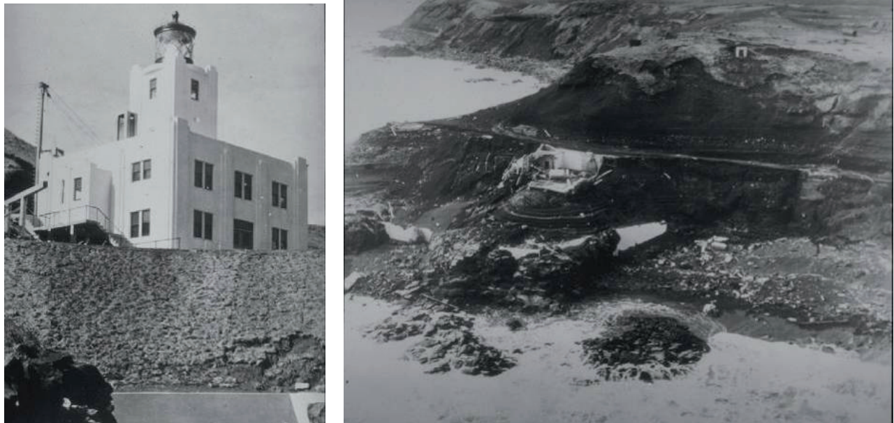
Figure 2-9 Scotch Cap Lighthouse destroyed by the 1946 Aleutian Tsunami.
